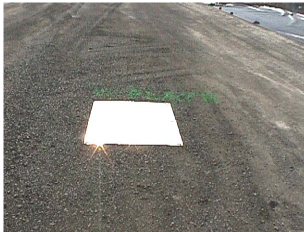
Figure 2. Copper plate under 21B layer in Section B.
