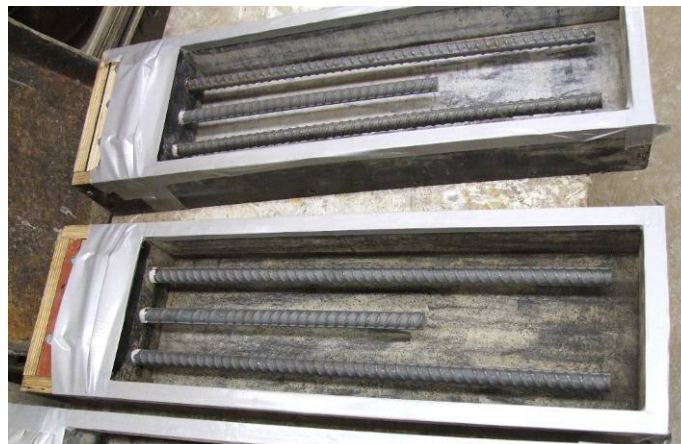
Figure 16. Photograph of tombstone molds that are ready for concrete casting phase.
