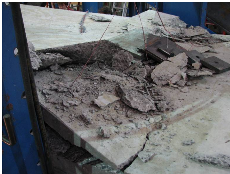
Figure 56. Crushing in the top of the deck
