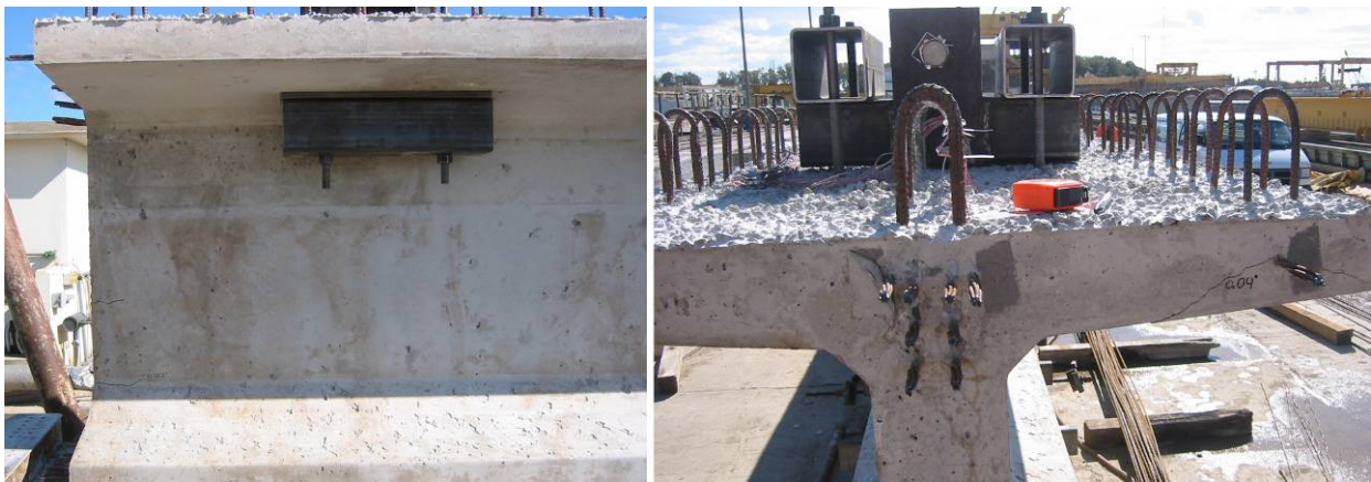
Figure 7. Girder lifting device
