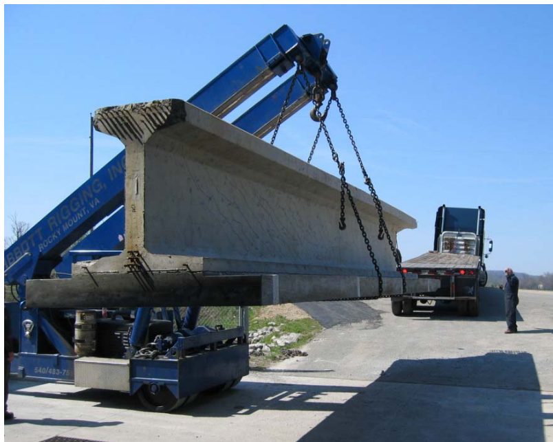
Figure 24. Removal of one half of the PCBT-53
