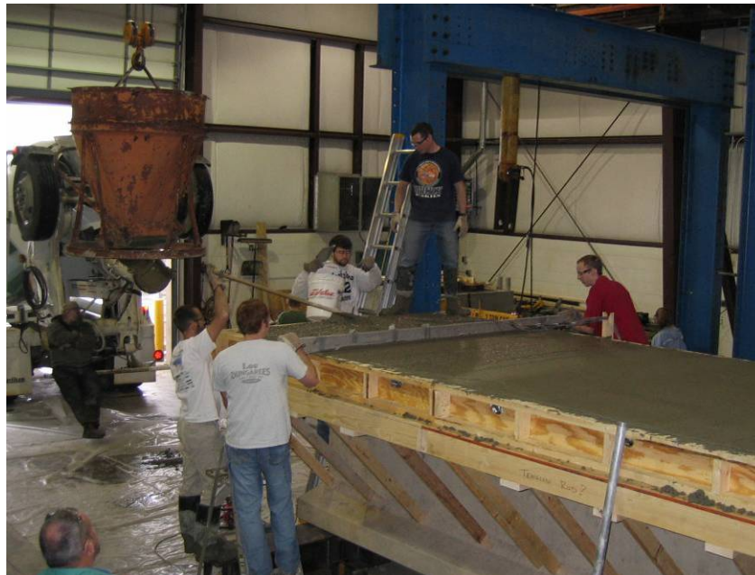
Figure 11. Deck concrete placement
