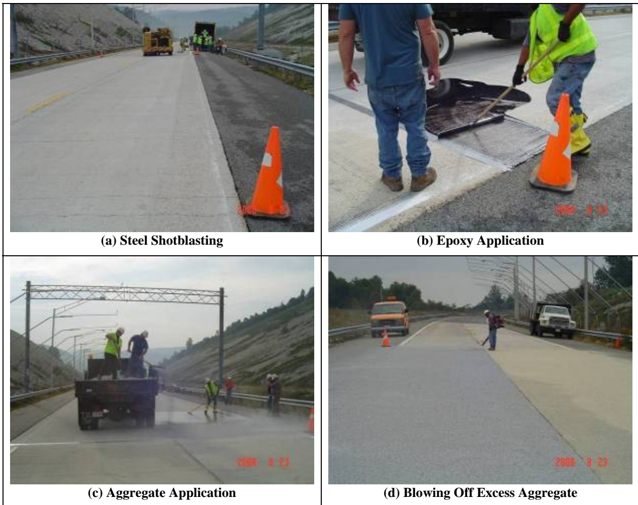
Figure 5. Summary of Construction Sequence at Smart Road
