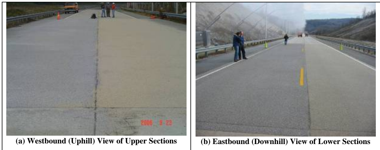
Figure 6. Side-by-Side Comparison of Overlay Systems at Smart Road. (a) VDOT Modified EP-5 overlay, (b) SafeLane overlay.
