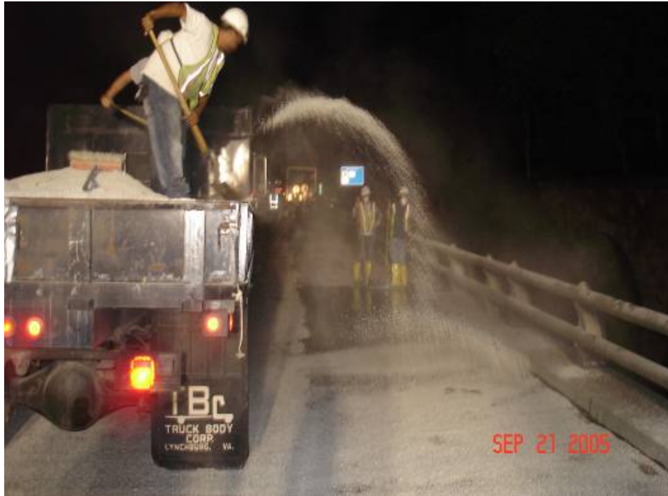
Figure 2. SafeLane Overlay Being Placed on Shoulder of I-81 Structure 2037
