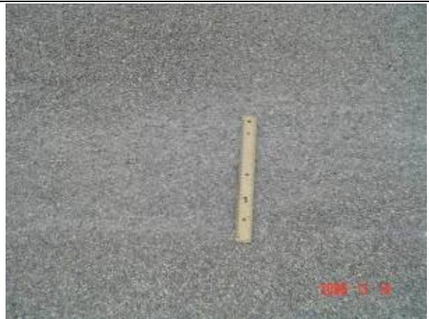
(e) Close-up of skid mark
