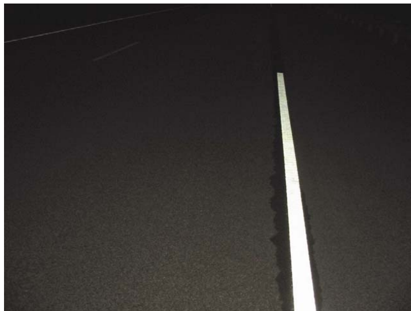
Figure 2. End of Pavement Marking on Asphalt
