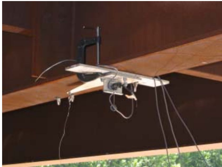
Figure 9. Deflectometer Clamped to Steel Girder
