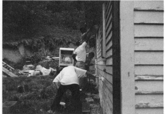
Tech Volunteers put the finishing touches on a home. They scraped and repainted the house for the elderly owner.
