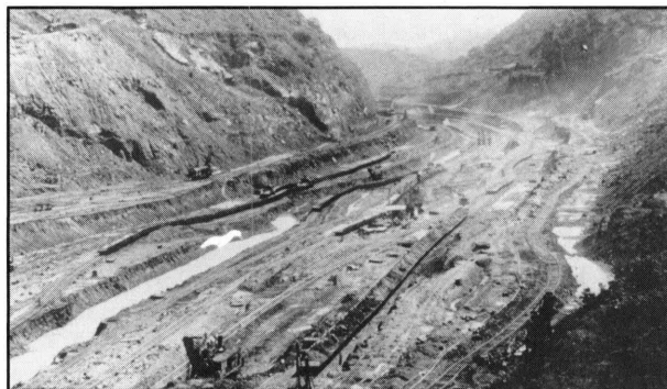
Construction of the canal through the Gaillard Cut, 1912.
