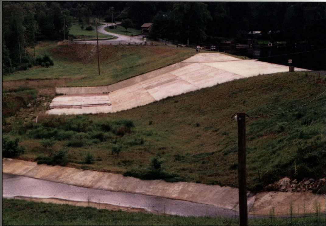
The Carter D. Martin dam, with a view of its spillway.
