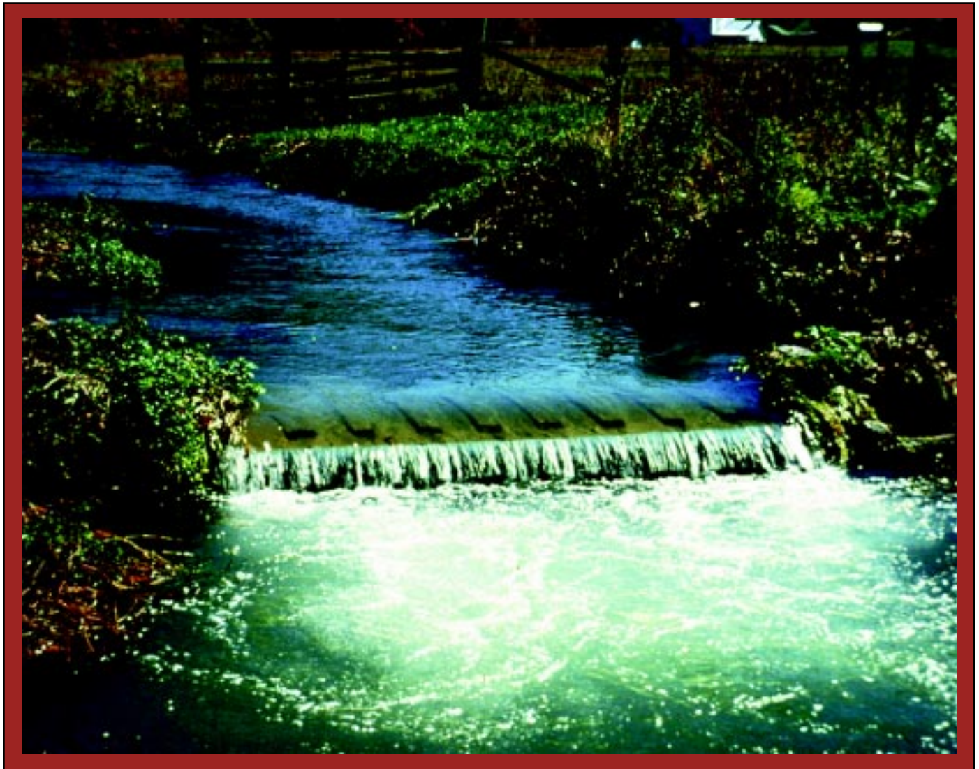
A pool former (low waterfall) is used to improve sportfish habitat by aerating the water and creating a downstream plunge pool.
