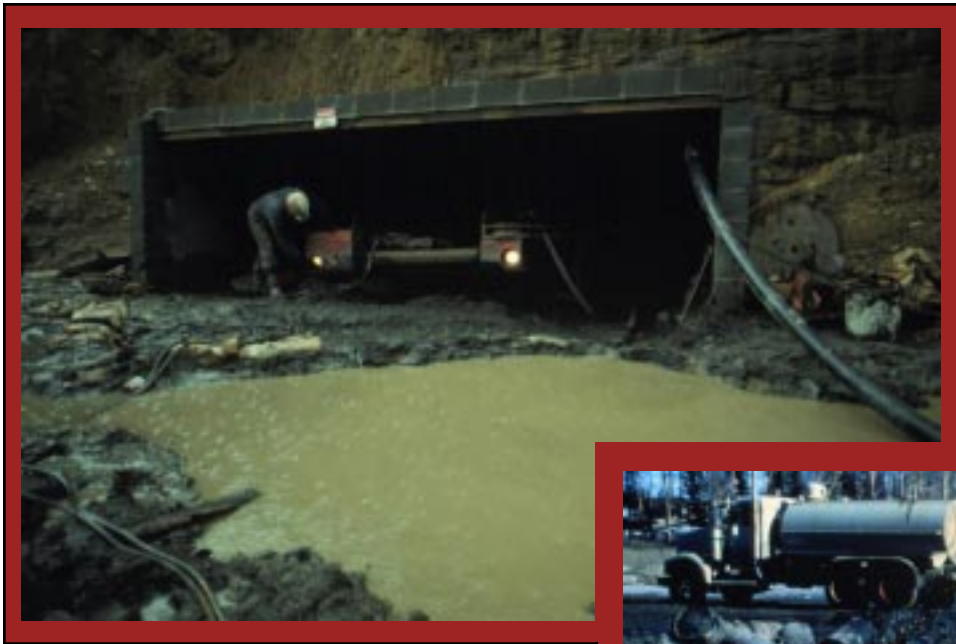
Coal silt runoff and deadly acids seeping from underground and surface mines pose major threats to stream water quality and aquatic life.
