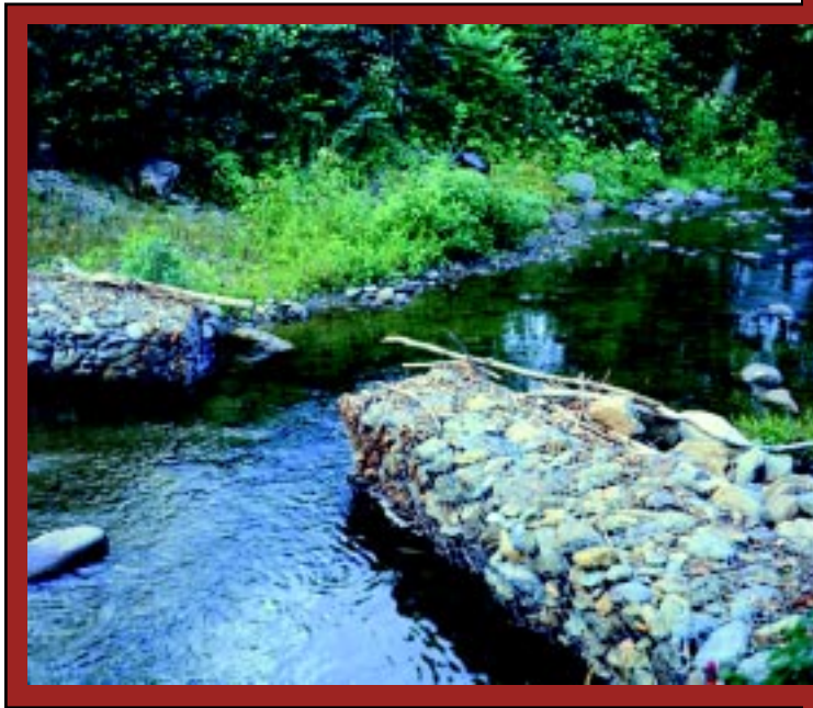
A pair of gabions (rock-filled wire cages), here used as wing deflectors, divert the current away from the banks, narrow and deepen the channel, and increase flow
