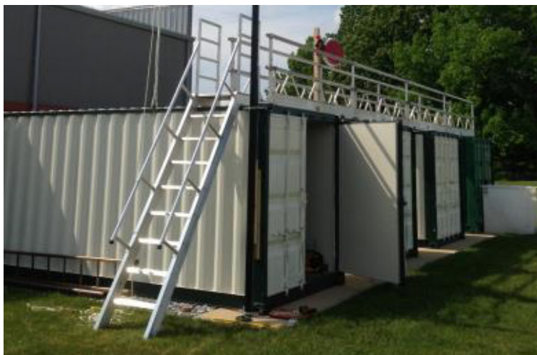
Figure 3-4: Inclined ladder for the competition. Image used with permission from DARPA, http://www.darpa.mil/NewsEvents/Usage.aspx , 2013.
