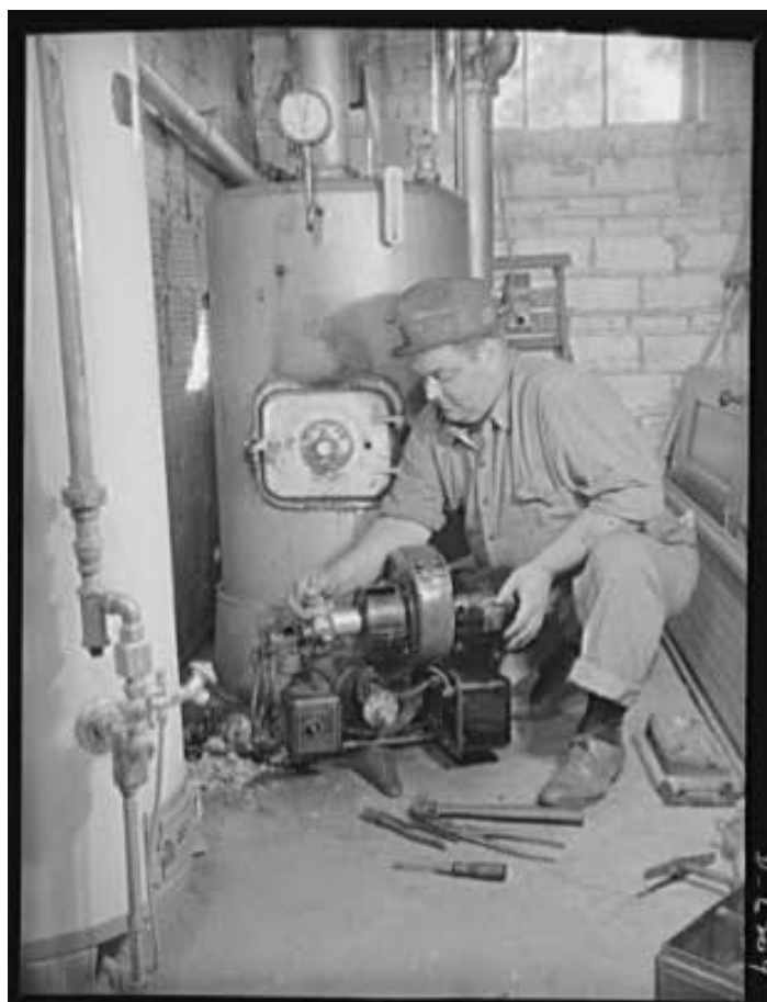
Figure 5: A maintenance man works to show how easy it can be to convert fuel-oil furnace to coal, 1942 (Library of Congress Prints and Photographs Division)
