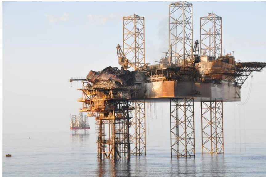
Fig. 2. Fire damage and structural collapse of the steel structure of an offshore platform off the coast of Australia [6]. [Fair use determination attached in Appendix C]
