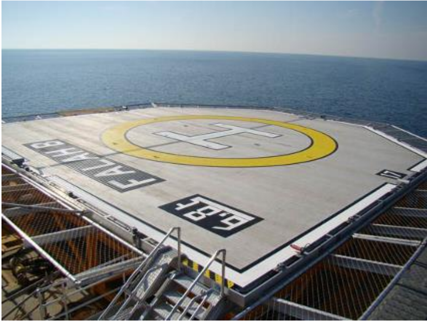
Fig. 1. Aluminum helicopter deck on offshore processing platform [1]. [Fair use determination attached in Appendix C]
