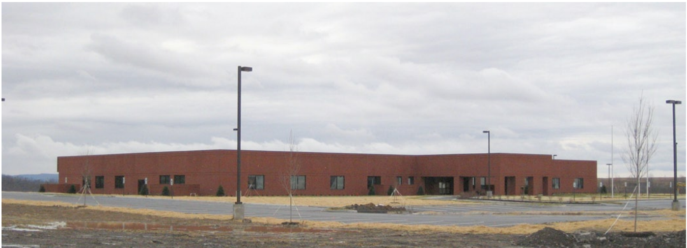
Figure 2. The Sykes Enterprises building at the Southern Gap Development Area in Buchanan County (see figure 1) in winter, prior to initiating operations. Because the site was compacted thoroughly and effectively during reclamation operations, the firm was able to install modern communications equipment that is sensitive to ground movement, as on a natural site.
