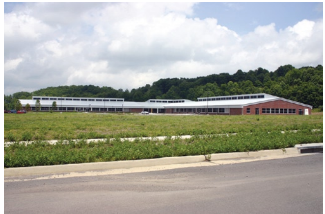
Figure 4. Lonesome Pine Technology Center, at Lonesome Pine Business and Technology Park in Wise County. This building was constructed on a reclaimed surface mine, as described in figure 3.
