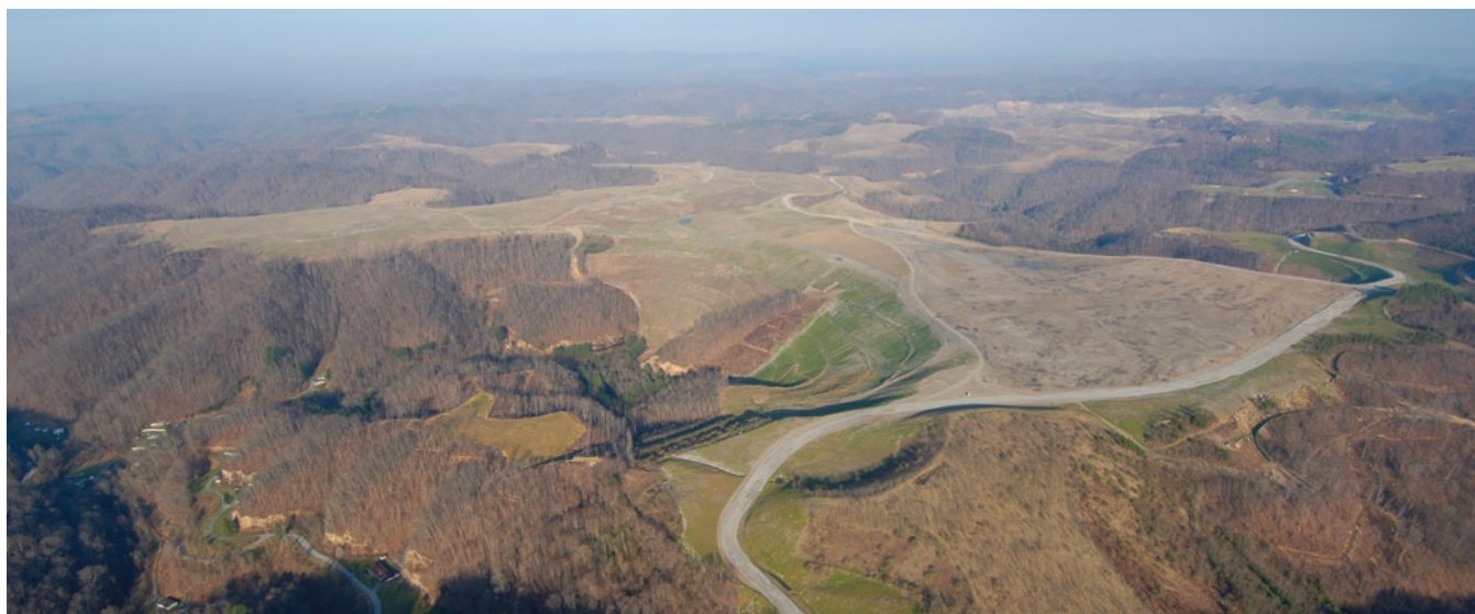
Figure 1. A portion of the Southern Gap Development Area in Buchanan County after reclamation but prior to building development. This site was prepared for industrial use by the mining and reclamation operations; thus, the spoil compaction and road development were cost effective. The paving and utility accesses necessary to enable the site to serve an industrial use were completed as a cooperative effort by the mining contractor and Virginia Coalfield Economic Development Authority (CEDA).
