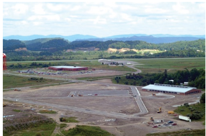
Figure 3. An aerial view of Lonesome Pine Regional Business and Technology Park in Wise County. Because the surface-mined site where the park is located was not compacted as needed to support industrial facilities during reclamation, the site was compacted to a more stable configuration after mining and reclamation were complete. The post-reclamation compaction operations are more costly and less effective than compaction that is applied during reclamation, when spoil and rock materials are being placed. Nonetheless, post-reclamation compaction operations were able to stabilize this mine site, and it now supports a variety of public and industrial facilities and operations.
