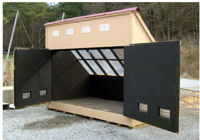
Figure 4. Rear view of kiln showing access doors.
