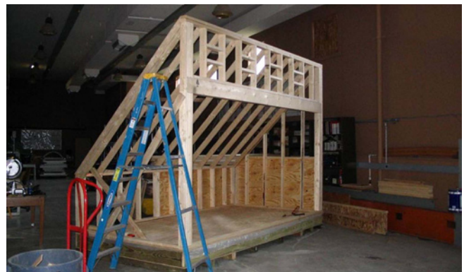
Figure 2. Interior framing showing fiberglass insulation.
