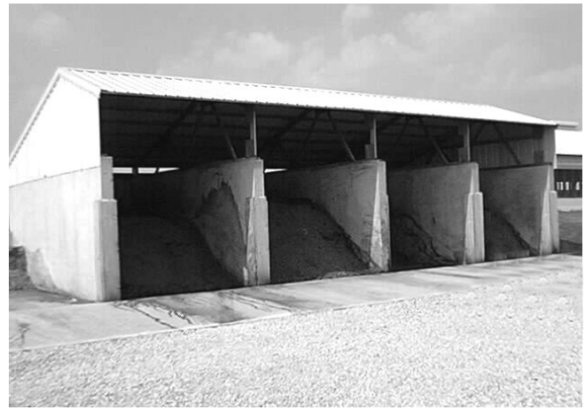
Figure 6. Structure constructed with both the floor and bin sidewalls out of formed concrete
