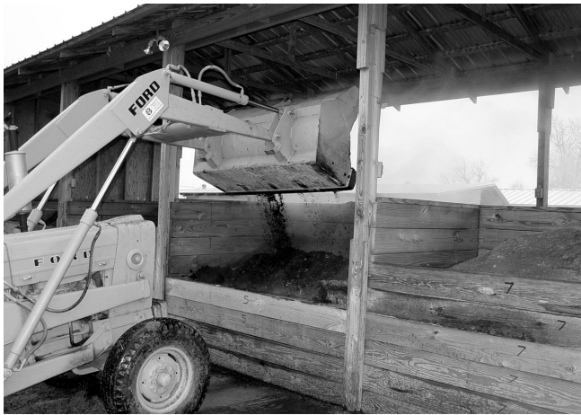
Figure 5. A pole-type structure with a concrete slab floor
