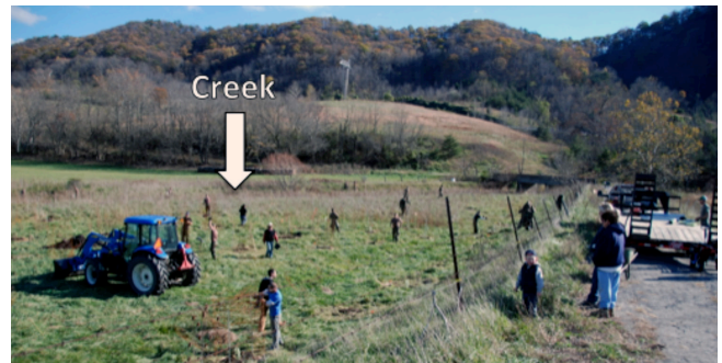
Figure 10. Virginia Tech students and Catawba community members plant and mulch trees and install deer protection in the riparian buffer.
