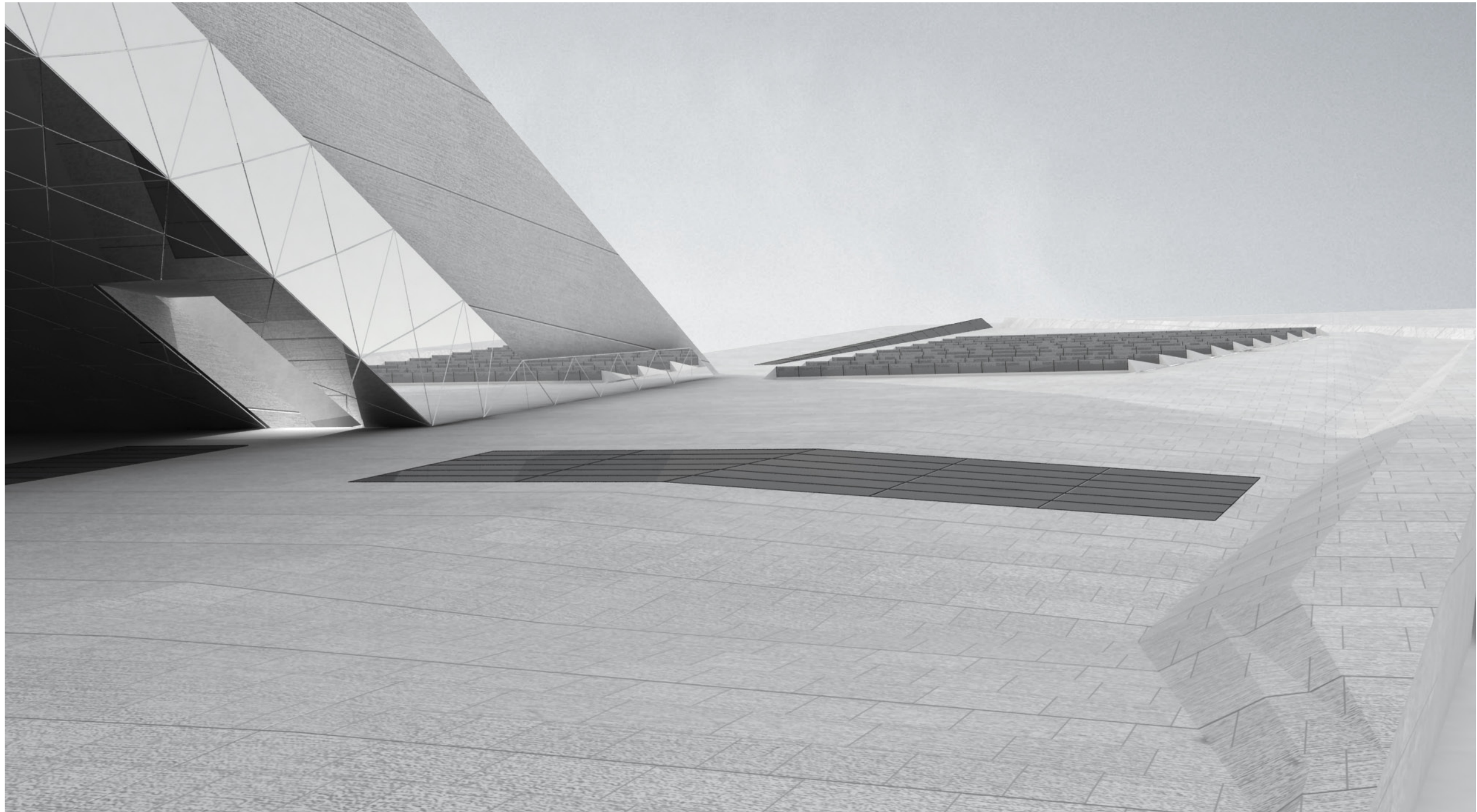
fig. 66 | The Roof top view
