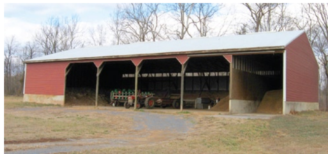
Figure 3. Permanently roofed storage structure
