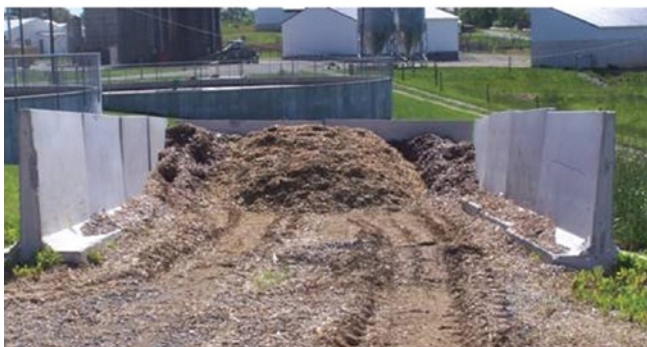
Figure 2. Bunker-type storage structure
