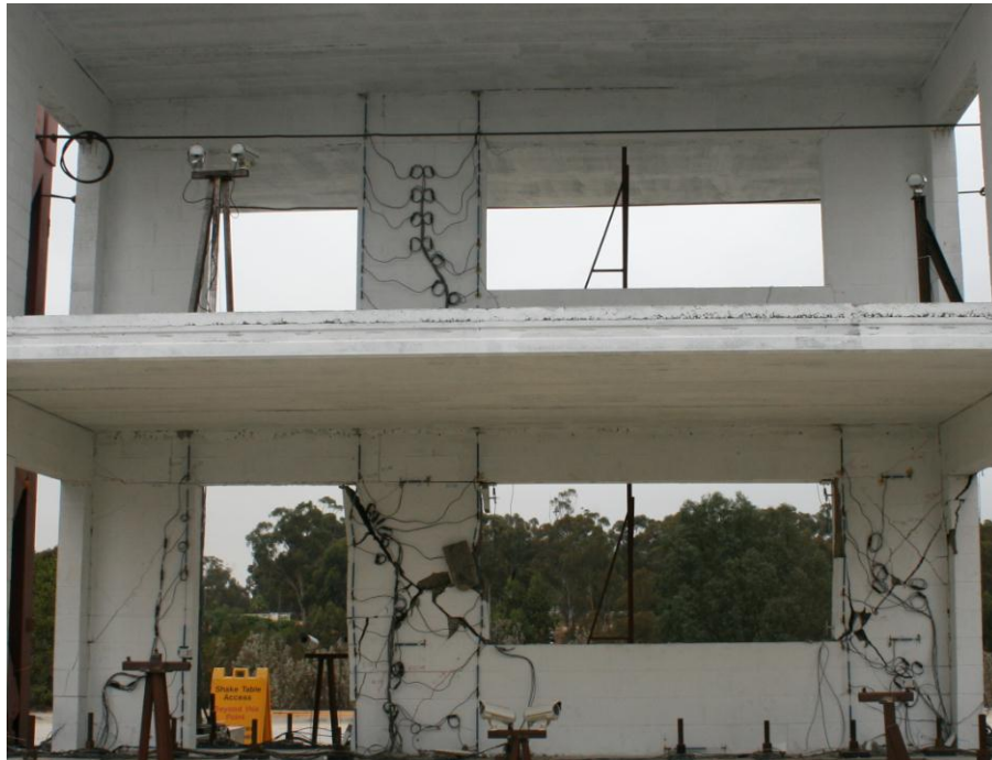
Figure 5.38: Structural Damage of Web Wall after Final Ground Motion. Mavros, M. 2013. Personal Communication. Used under fair use, 2014.
