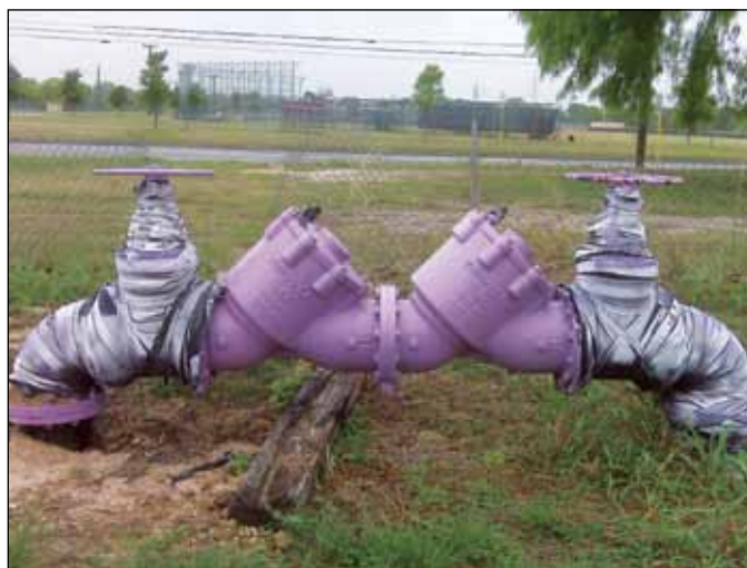
Figure 3-2. RPZ backflow prevention device. Source: EC Design Group, LTD.
