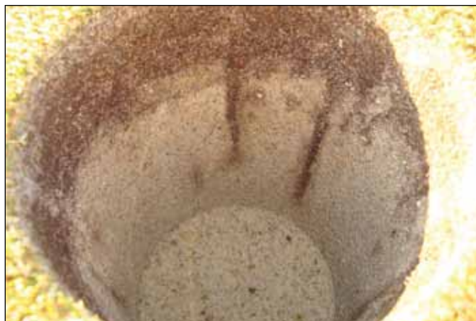
Figure 7-9. Results of high pressure water injection.
