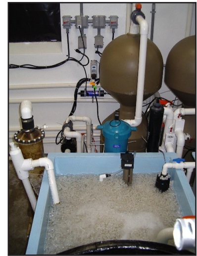
Fig. 1. RAS water treatment
