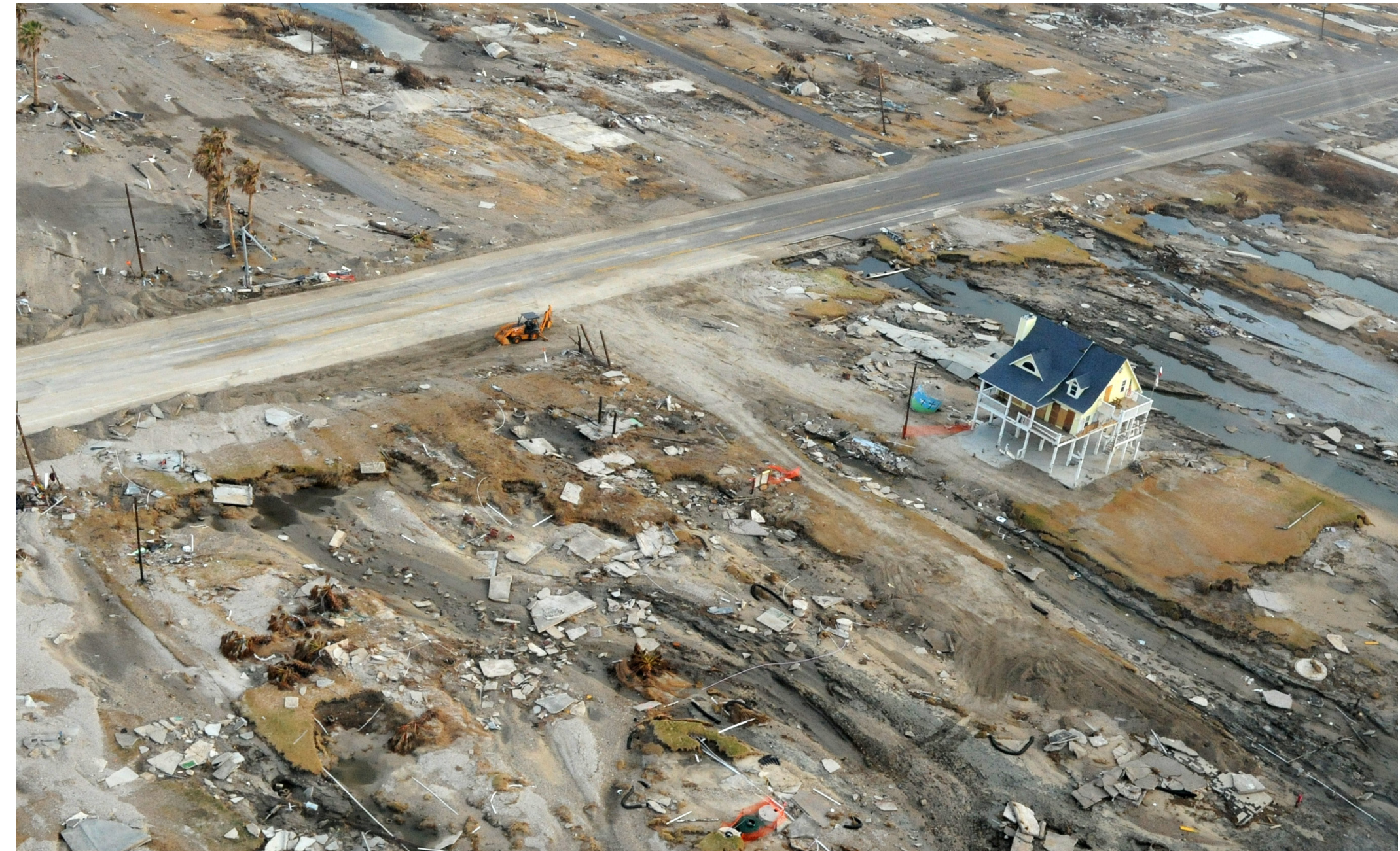
damage in gilchrist
