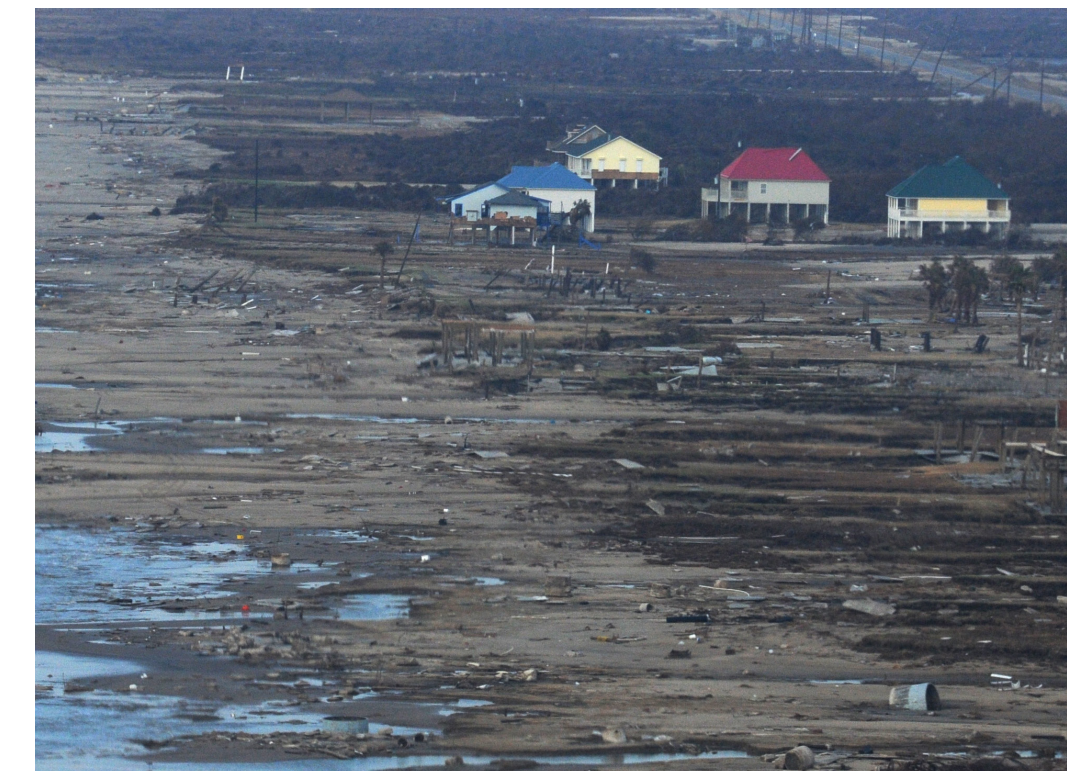
damage in gilchrist
