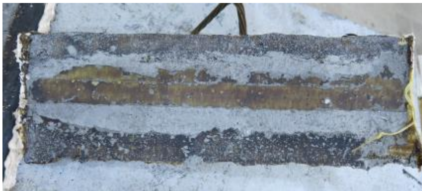
Figure 63: Picture of debonded, intact Kevlar reinforcement
