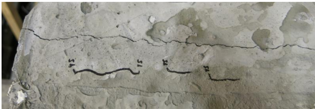
Figure 102: Crack on top of the first specimen after failure
