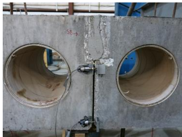
Figure 41: Picture showing instrumented joint
