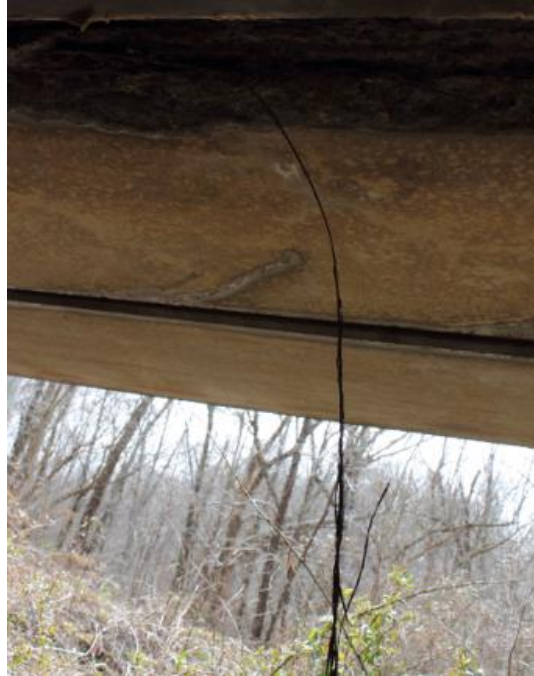
Figure 4: Corroded prestressing strand hanging from large concrete spall near a shear key
