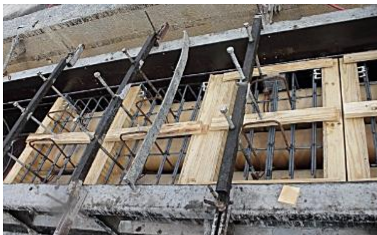
Figure 11: Voided slab forms sitting in prestressing beds
