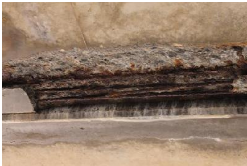
Figure 3: Concrete spalls, corroded prestressing strands, and staining under a shear key
