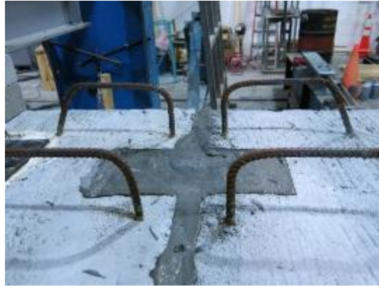
Figure 20: Picture of cured UHPC joint
