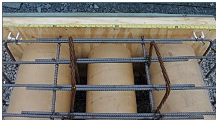
Figure 10: Voided slab formwork and rebar cage
