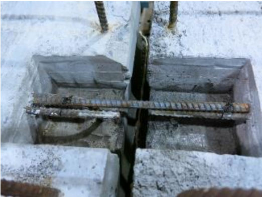
Figure 19: Picture of Blockout with tied in lap splice bar before UHPC placement
