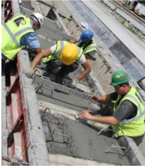
Figure 13: Workers applying finishes to the concrete
