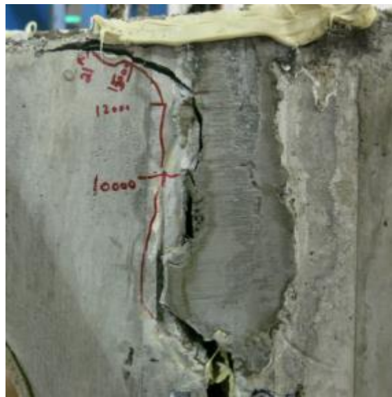
Figure 73: Picture showing the cracked south shear key of specimen 3
