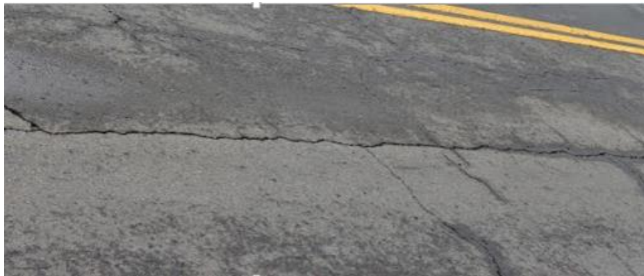
Figure 2: Longitudinal Reflective Cracking in asphalt overlay
