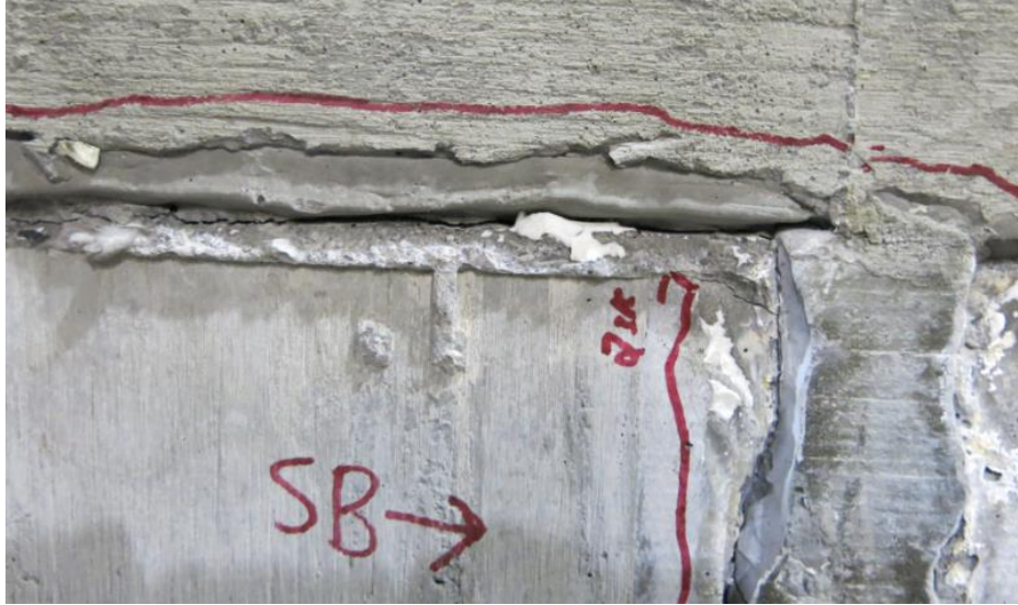
Figure 92: Close up showing cracking along topping voided slab interface
