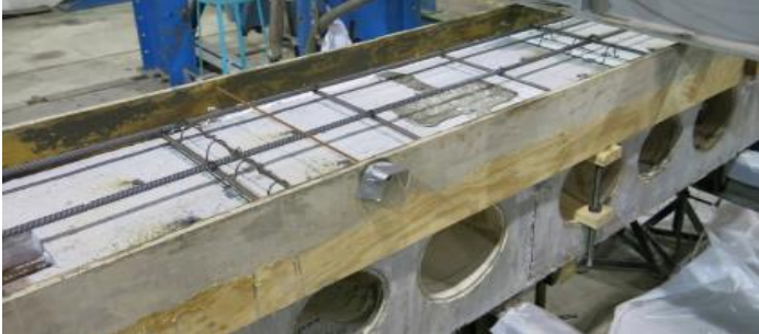
Figure 23: Picture showing reinforcement mat in place and formwork for concrete topping
