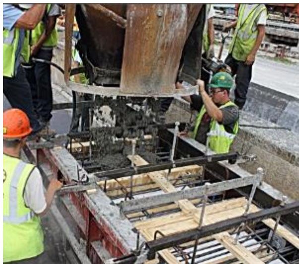
Figure 12: Concrete being poured from the skip
