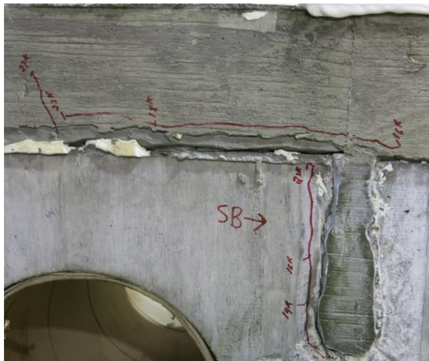
Figure 91: South joint showing typical cracking pattern observed during final static test
