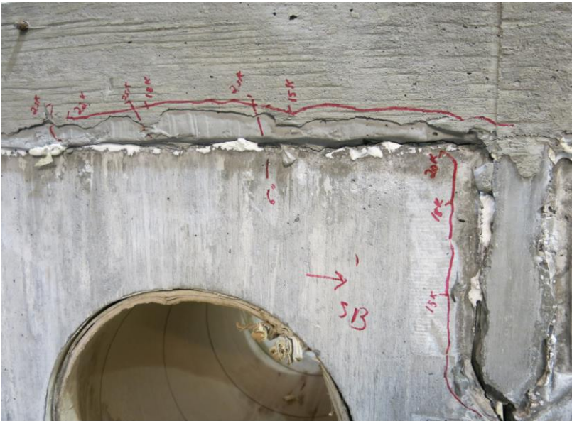
Figure 98: Typical cracking pattern for specimen 6 key
