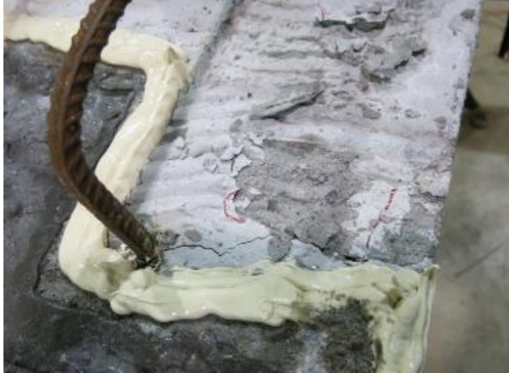
Figure 74: Picture of concrete crushing and concrete spalls on top of specimen 3
