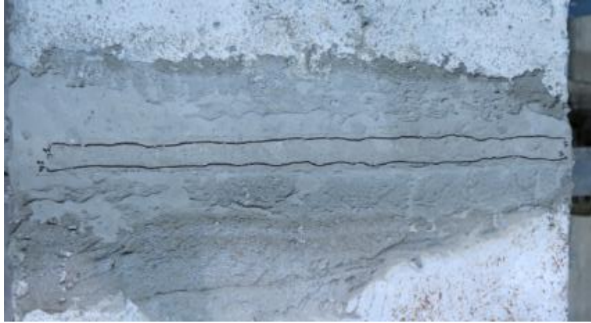
Figure 65: Picture showing marked shrinkage cracks before placement of the Kevlar
