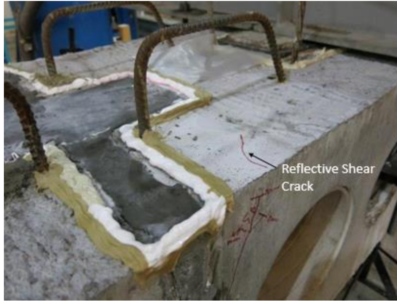
Figure 83: Picture showing reflective cracks on the middle section near the south joint
