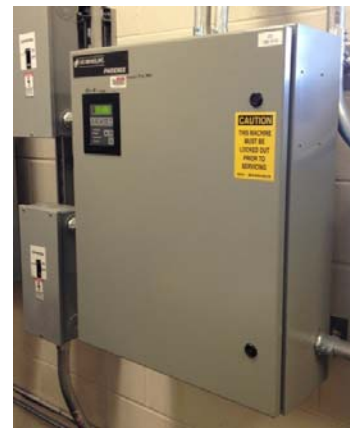
Figure 8 – Prime mover variable frequency drive
