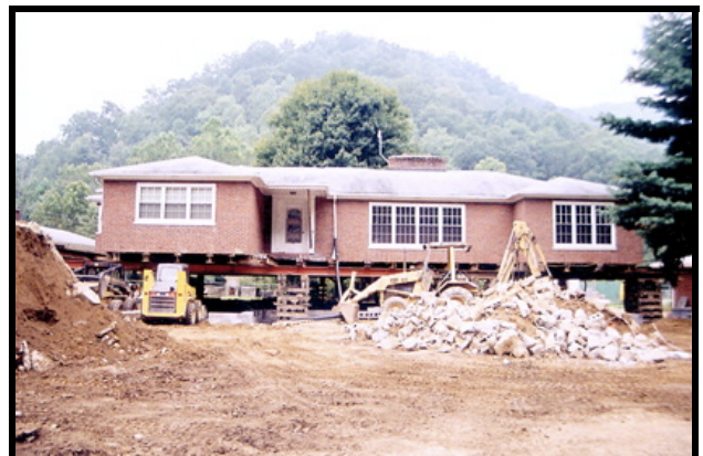
House elevation in Grundy as part of the town's flood-protection project. (Photo from Virginia Mountaineer , September 1, 2005, reprinted with permission.)
