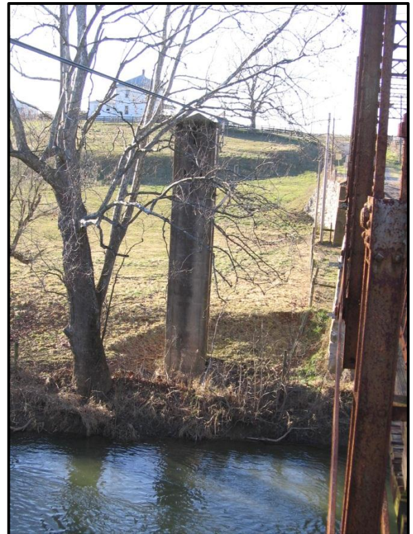
Stream-gaging station on the Middle River at Mt. Meridian (Augusta County), 12/16/09.
