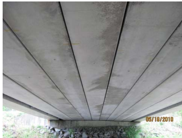
Figure 1-8 Adjacent box beams of New York Pilot Bridge (Rutgers University 2009)
