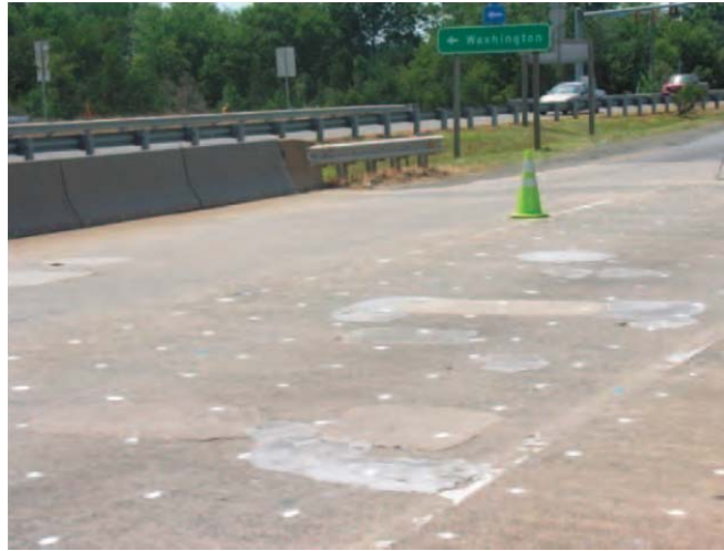
Figure 1-3 Deterioration on Virginia Route 15 Bridge (Photograph by Gucunski et al.)
