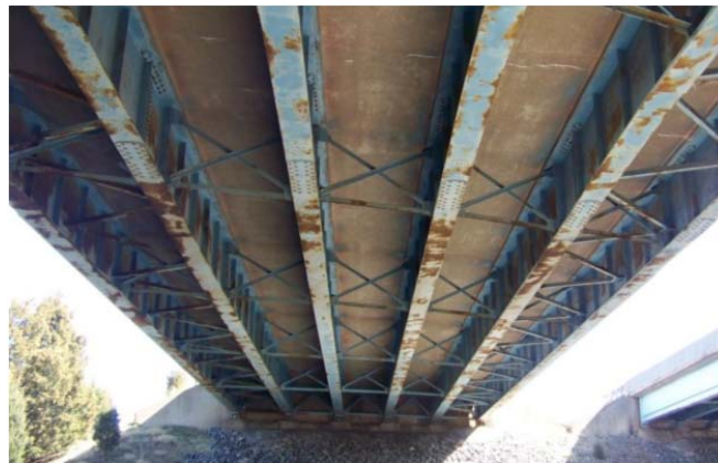
Figure 1-2 Virginia bridge girders and cross frames (Photograph by Collins)
