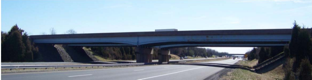
Figure 1-1 Virginia Route 15 Bridge over Interstate 66 (Photograph by Collins)
