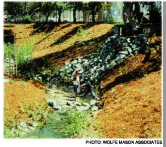
Figure 5. Blackberry Creek after construction
