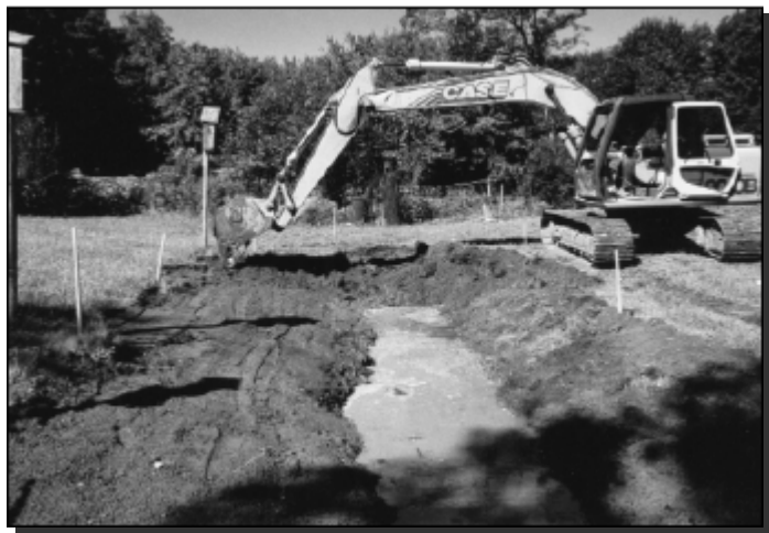
Figure 14. West Ox Pasture Brook during daylighting
