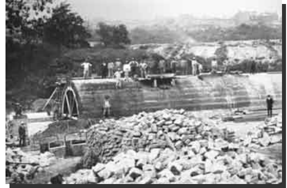
Figure 2. Wingohocking Creek Sewer under construction. 1909
