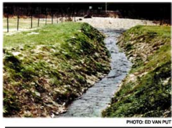
Figure 9. Darbee Brook post-daylighting
