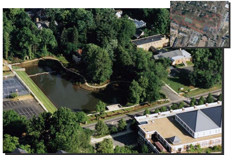
Figure 12. Sedimentation basin at “The Dell” pre- and post-construction
