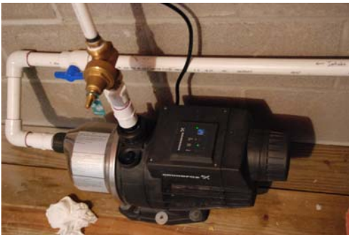
Figure 7. Grundfos 800 watt rainwater pump
