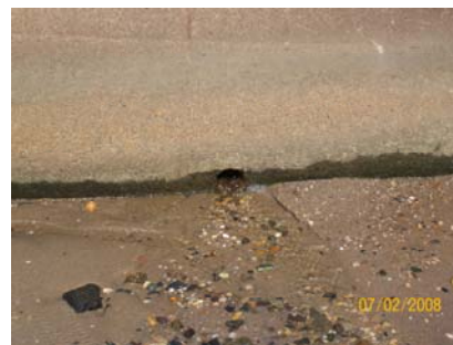
Beach Drain Pipe Hole
