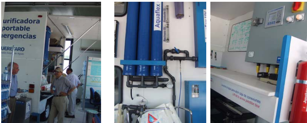
Figure 8. Emergency water processing unit in Querétaro
