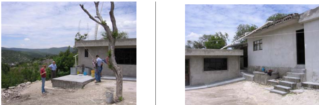
Figure 7. Rooftop rainwater collection and water delivery in Xacxamayo
