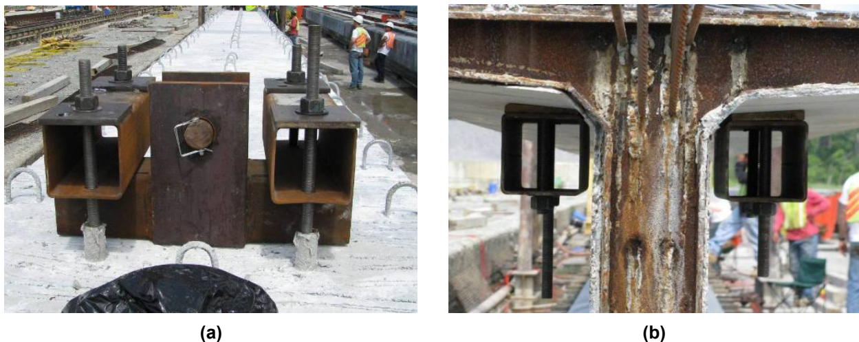
Figure 3-6. (a) Top and (b) Bottom of special lifting device used for PCBT-45 beams in this study.
