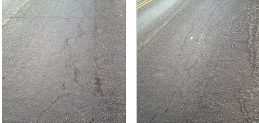
Figure 11. South Franklin Street Local Premature Cracking (May 2014)
