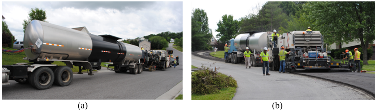
Figure 9. Recycling Equipment, (a) Front View, and (b) Back View, Photos by Todd Walters, 2013, Used with Permission
