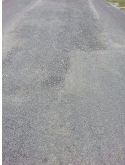
Figure 14. Miller Street (August 2013): After Recycling, before HMA Overla
