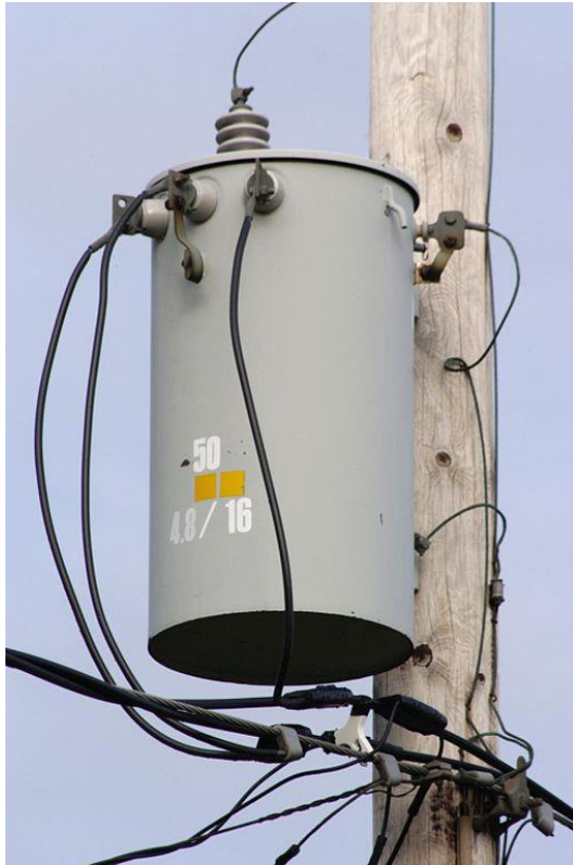
Figure 4: Single-Phase Pole-mount Distribution Transformer. Sources: "Transformers," [Online]. Available: http://en.wikipedia.org/wiki/Transformer . [Accessed 19 February 2014]. "Inside an electric distribution transformer," [Online]. Available: http://waterheatertimer.org/See-inside-main-breaker-box.html . [Accessed 9 April 2014]. Used under fair use, 2014
