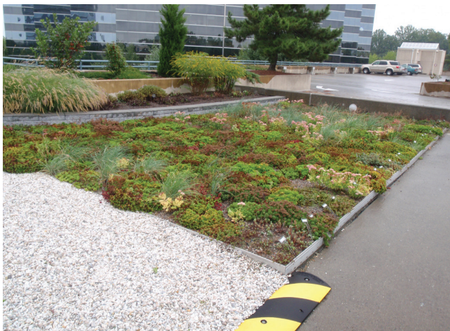
Figure 1. Photograph of vegetated roof. Note that roof contains both intensive and extensive sections.
