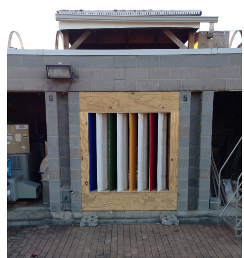
03/05/2014 Installation of the color reflectors
