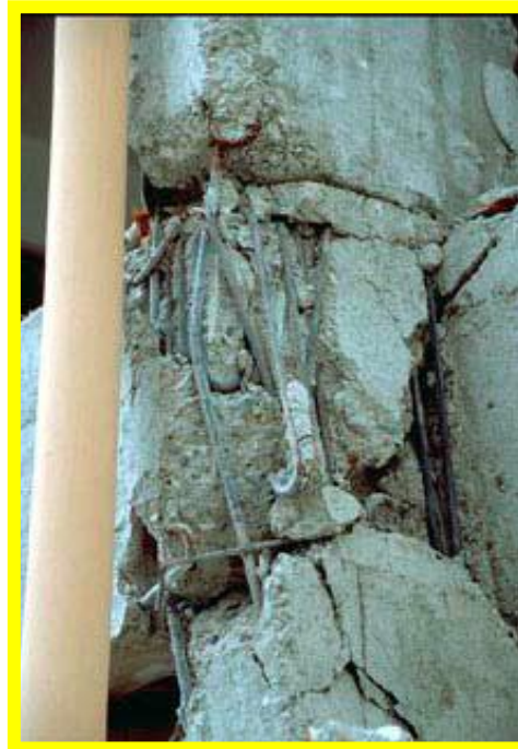
b) Close up of beam-to-column joint failure
