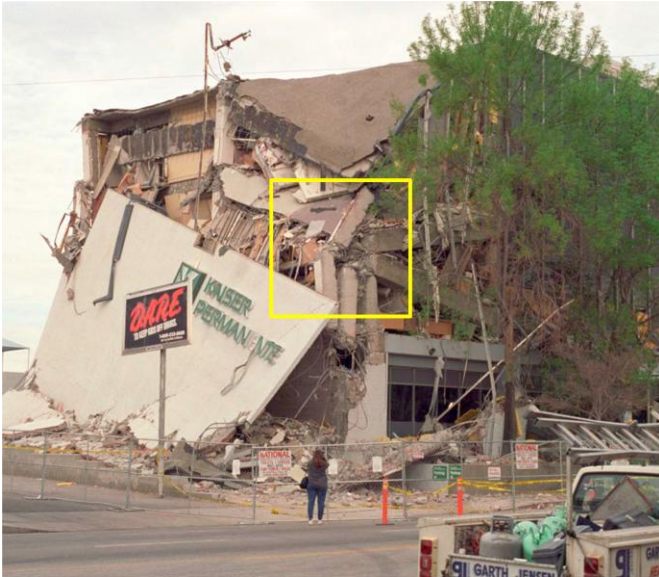
a) Partial building collapse
