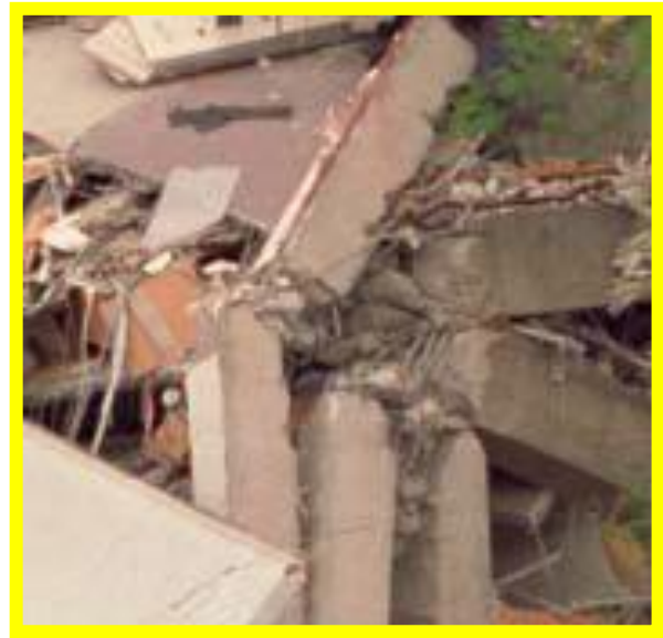
b) Close up of beam-to-column joint failure
