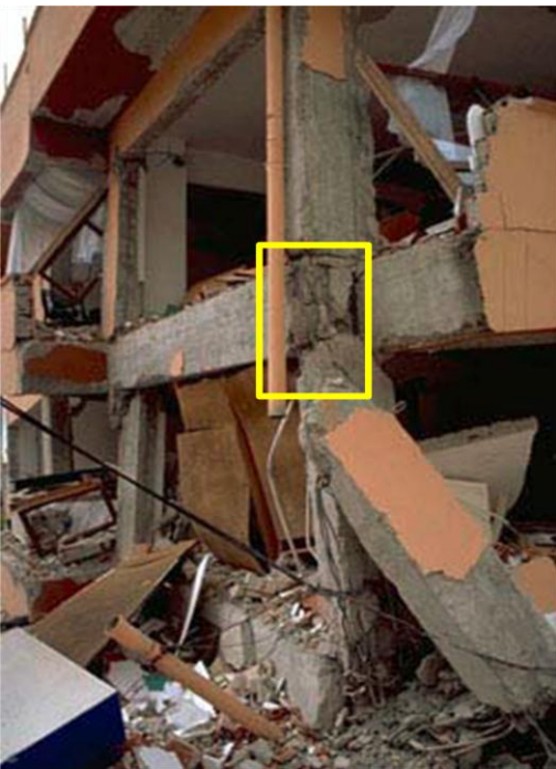
a) Partial building collapse
