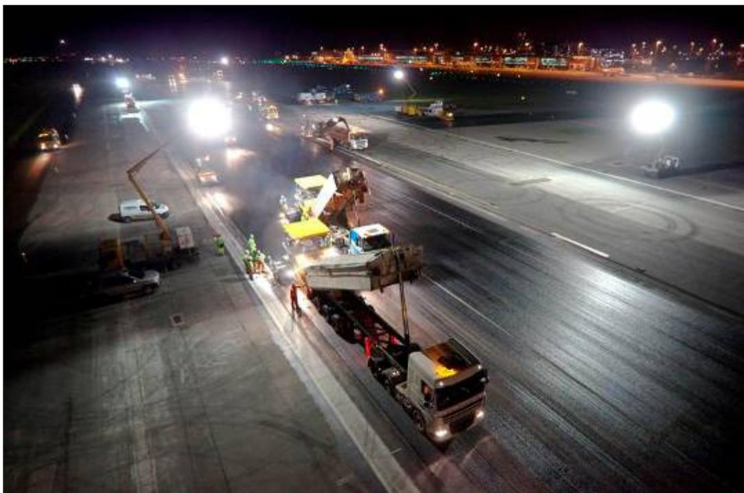
Figure 6 – Laying and compaction of BBA surface course at Manchester Airport (Courtesy of Costain) [11]
