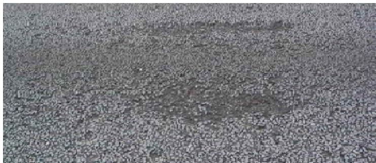
Figure 7 - Example of surface disintegration on hot rolled asphalt.
