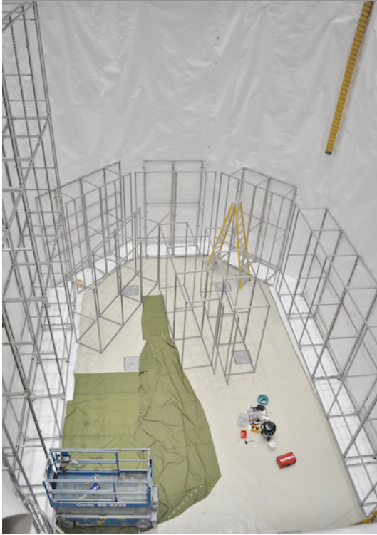
(a) Assembly of OWS with unistrut.
