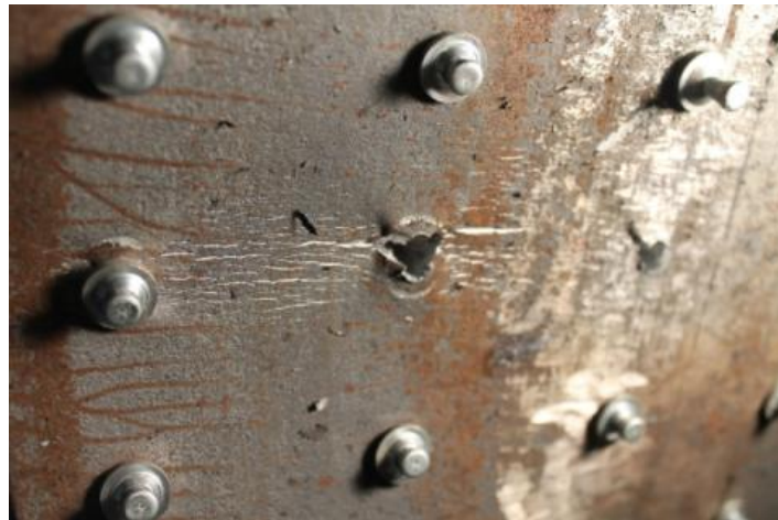
Figure 3.62 – Cracks Forming on the Surface of the Bottom Flange for Specimen 12 (W36x150 with no RBS and Grid of PAF)
