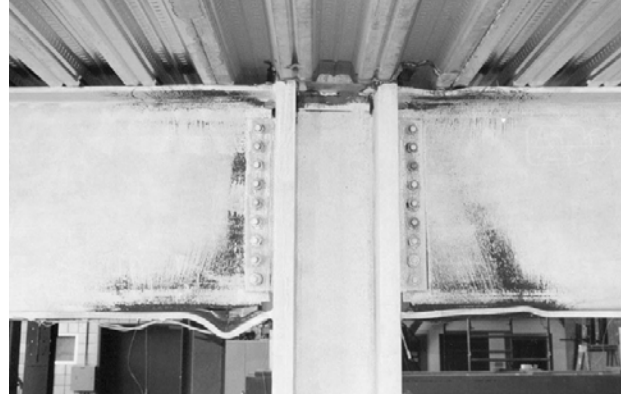
Figure 1.2 - Picture of Beam-to-Column Connection Test with Welded Shear Studs and Composite Floor Slab After Testing (Picture from Uang et al. 2000).
