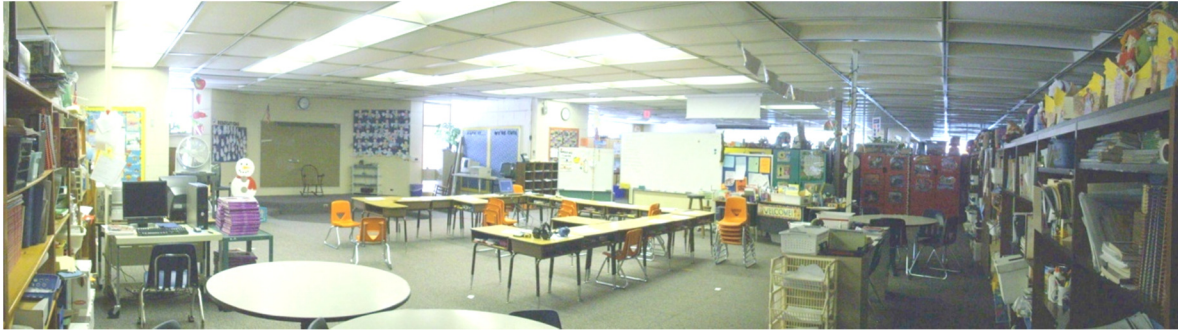
Figure 19. Partial height partitions separate this classroom from adjacent classrooms. Note the daylight coming over the far wall in the image
