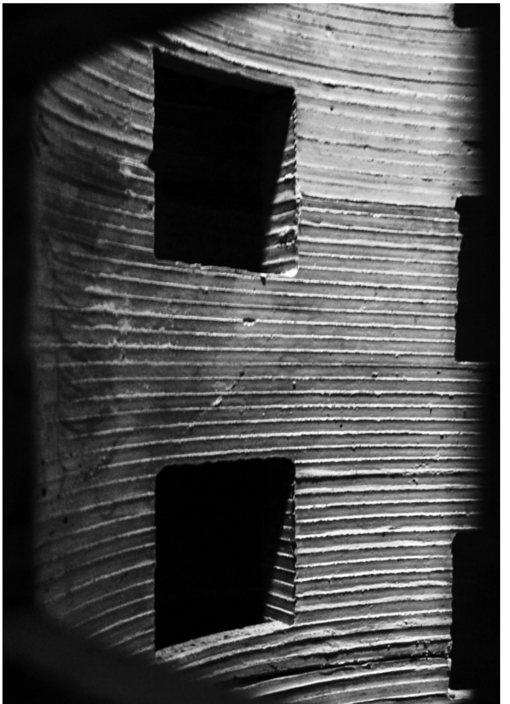
from top: front view; interior view of the open shaft
