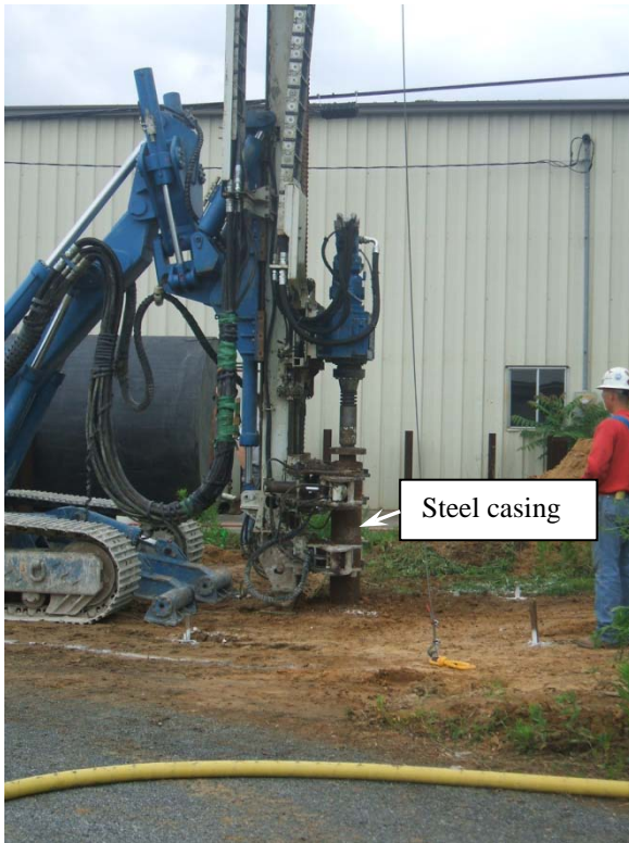
(a) positioning drill rig
