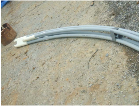
(a) Cylindrical spacers for the U-tube
