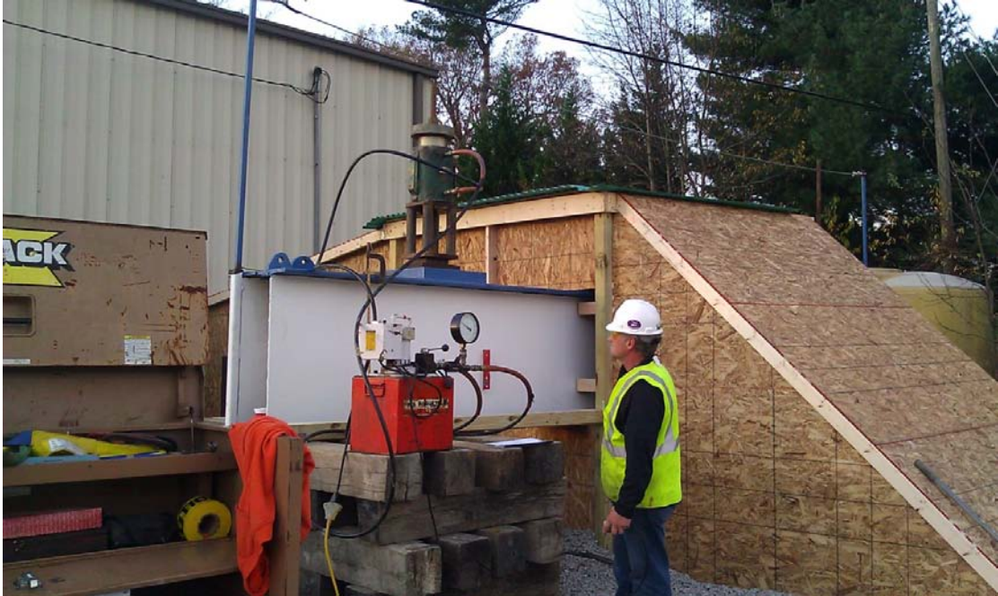
(b) Tensioning of the reaction piles
