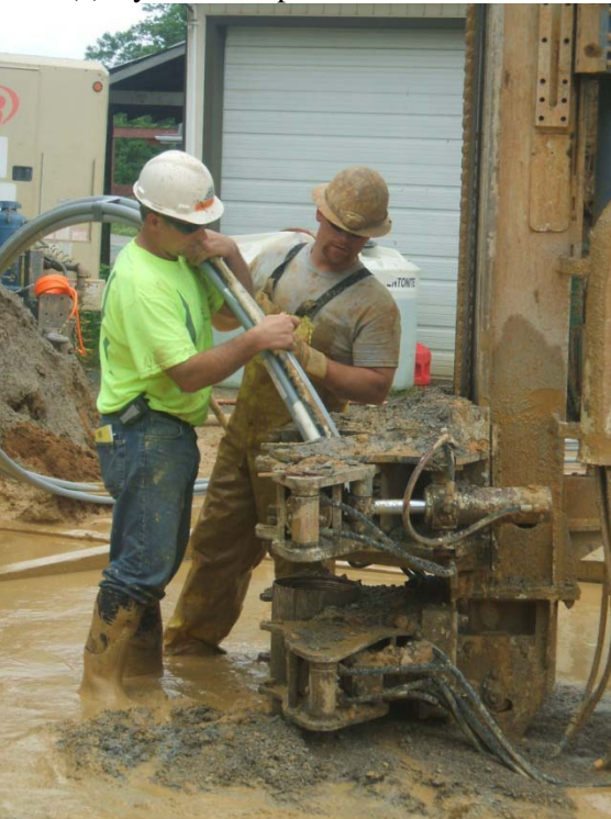
(b) tube installation
