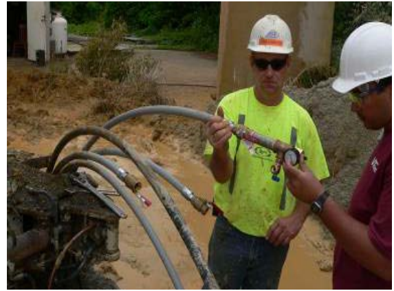
(c) pressure testing
