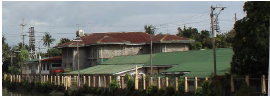
Hospicio de San Jose located on Convalencia Island across the Pasig River
