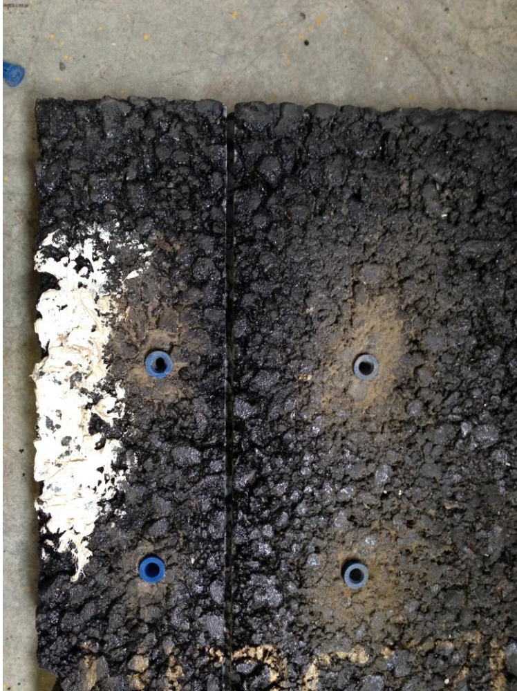
Figure 4 Slab with a Crack
