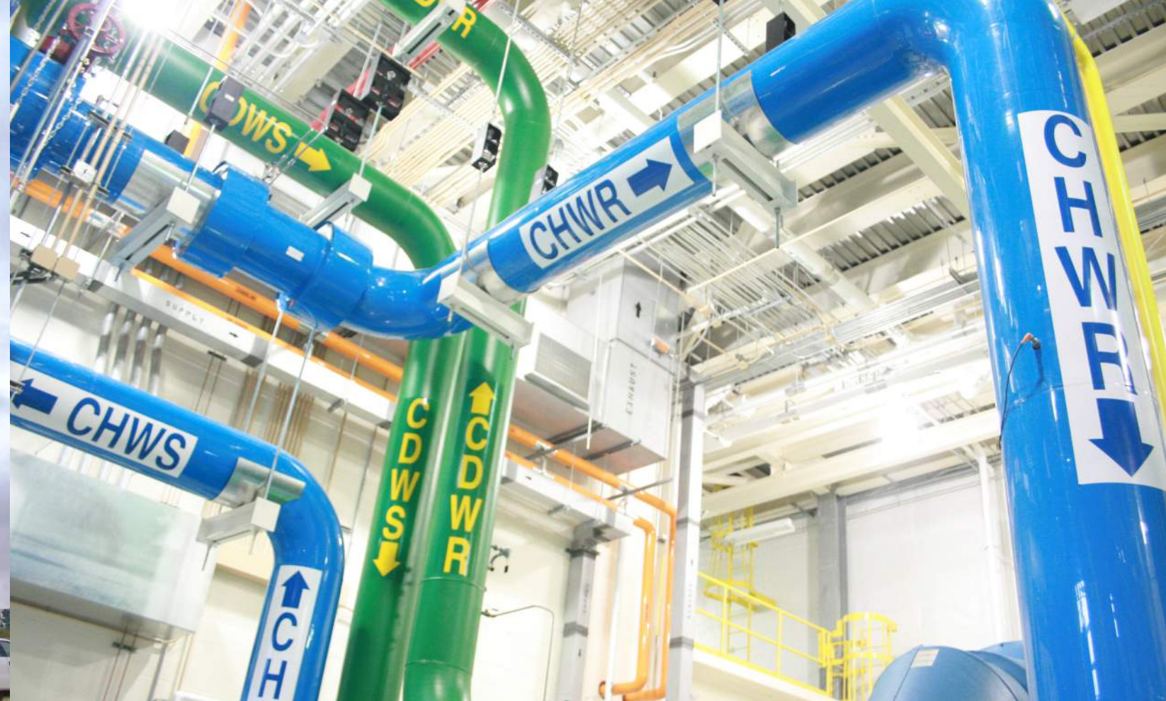
View of piping system just above chillers. Labels indicate the type and direction of water in the pipes.
