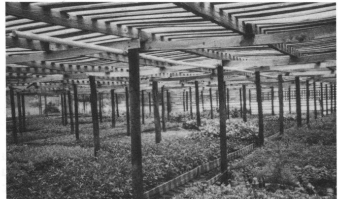
Liner production in a lath house. Lath should run north and south to provide alternate shade. (Gresham's Nursery, Richmond, VA, no longer in business)
