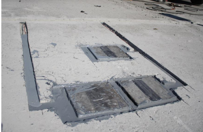
Figure 128. Photo. Pouring the epoxy in the prepared pits and cable trench.
