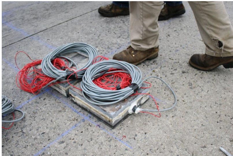
Figure 118. Photo. Marking the pavement for the alignment of the energy harvesters.
