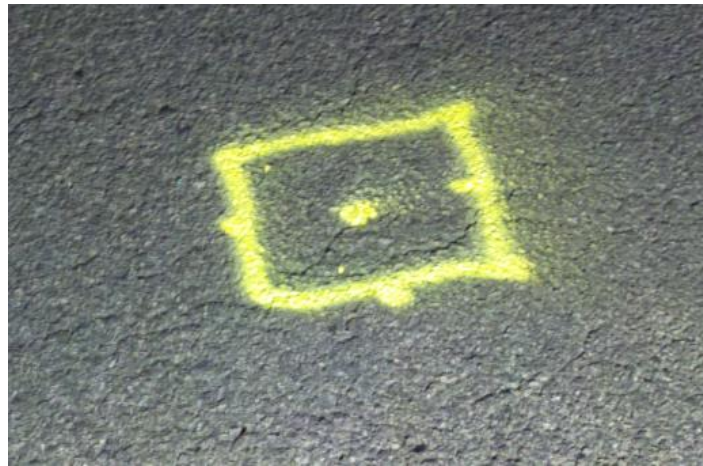
Figure 103. Photo. The pavement marked with the dimension and the location of the energy harvester.
