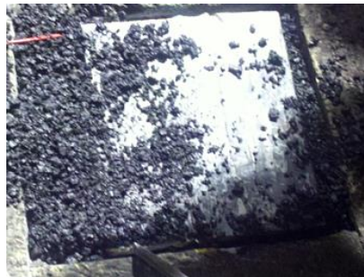
Figure 105. Photo. The energy harvester being covered with HMA.
