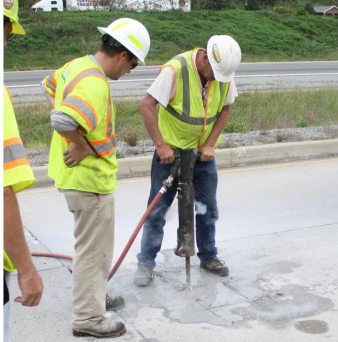
Figure 120. Photo. Jack hammering the cut pavement.
