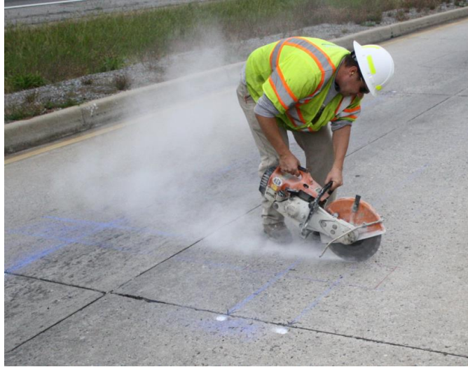
Figure 119. Photo. Cutting holes on pavement for energy harvesters.
