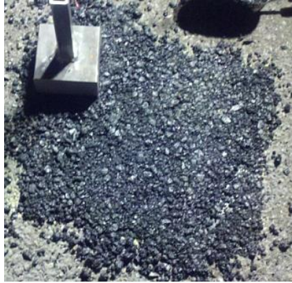
Figure 106. Photo. The energy harvester covered with slightly compacted HMA. A channel from the harvester to the shoulder was cut using the asphalt saw to place the electrical cord. The cord was covered with a protective PVC tube on the shoulder end. Figure 107 shows the cord covered with protective tube.
