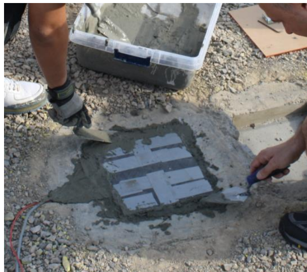
Figure 88. Photo. Filling the space with cement grout. As shown in Figure 89, two metal plates were placed on the harvester and the top of the metal plate was flush with the ground surface.
