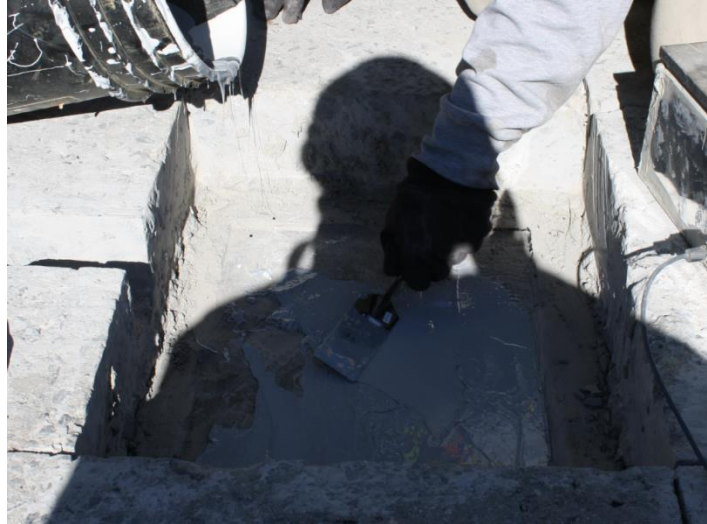
Figure 126. Photo. Applying a thin layer of epoxy in the prepared pits (to have a good bonding).
