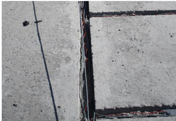
Figure 124. Photo. Cables in the prepared trench.
