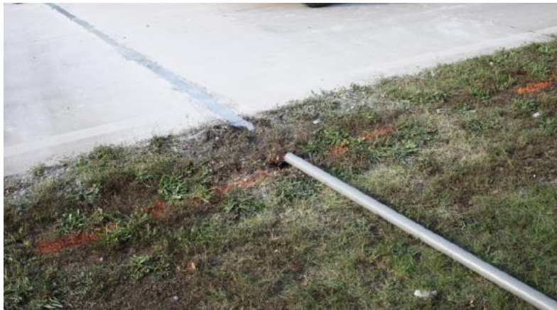
Figure 129. Photo. The protective conduit.
