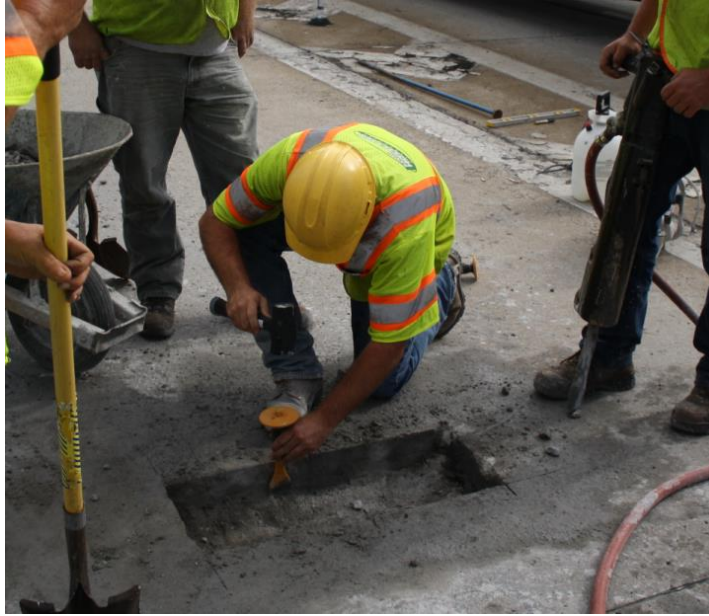
Figure 121. Photo. Chiseling out the remaining material and preparing the side wall and bottom.
