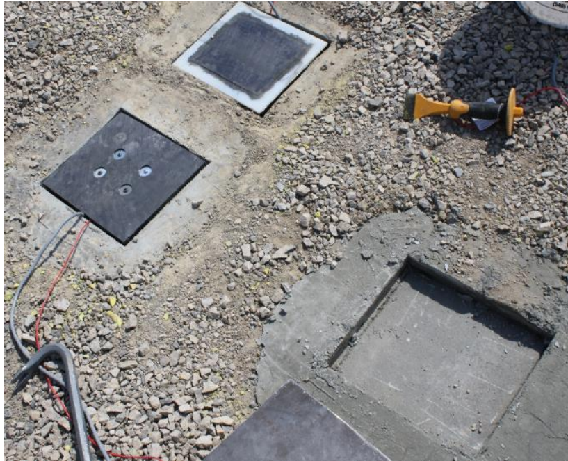
Figure 87. Photo. The energy harvesters in the ground without filling the space. The space between the harvesters and pit edges was filled with cement grout as shown in Figure 88. After the cement is set, no movement of the harvester would be allowed.
