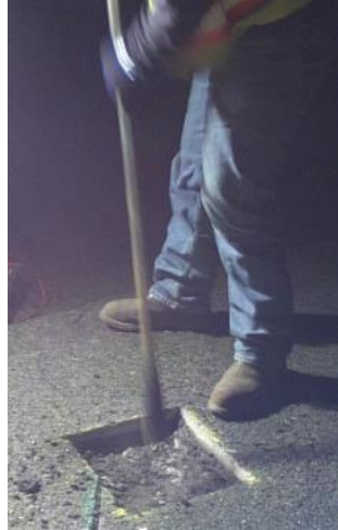
Figure 104. Photo. The scene of chiseling the pavement
