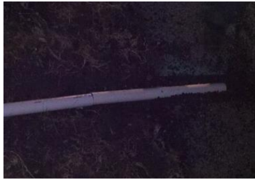
Figure 107. Photo. The electrical cord covered with a PVC tube. The 1.5-inch asphalt overlay was paved above the existing pavement lastly. Voltage output was measured after a two-day cooling phase.
