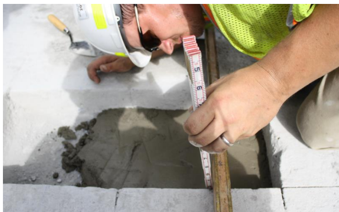
Figure 122. Photo. Preparing the bottom of the pits.
