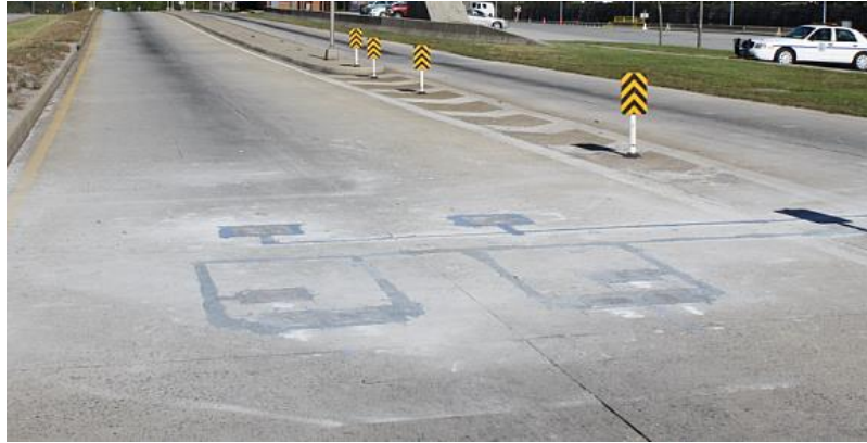
Figure 132. Photo. Final pattern of the eight energy harvest devices installed in the wheel paths of the bypass lane.
