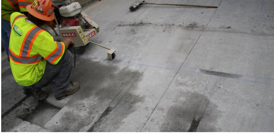
Figure 123. Photo. Marking the pavement for the cable trench.
