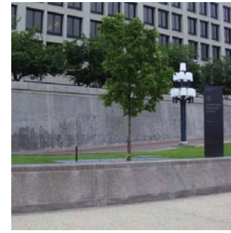
THE DOUBLE STARK WALLS ARE REDUNDANT FOR VEHICULAR PROTECTION AND DEPRIVE PEDESTRIAN USE OF THE INTERVENING SPACE
