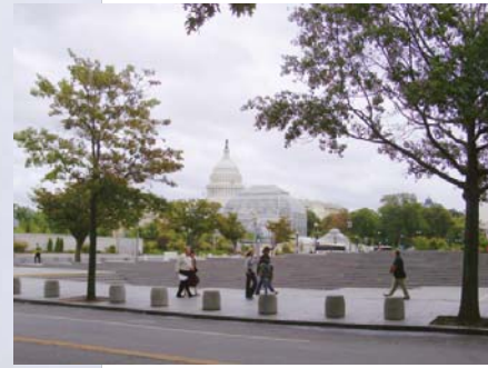
INSUFFICIENT HEIGHT BOLLARDS - PROVIDE LIMITED PROTECTION - VULNERABLE TO VEHICLES WITH HIGHER GROUND CLEARANCE - UNLIKELY TO ARREST VEHICLES PROGRESS AT BOLLARD LINE
