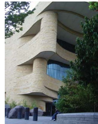
USE OF LANDSCAPE ELEMENTS BEGINS TO MORE EFFECTIVELY INTEGRATE THE SECURITY DESIGN HOWEVER THE BOLLARDS COULD EASILY HAVE BEEN DISPENSED.
