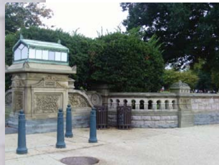
INTRODUCTION OF BOLLARDS IS AT LEAST RESTRAINED BUT MANHOLE MIGHT PROVIDE COMPROMISING ACCESS TO BOLLARDS FOOTING.
