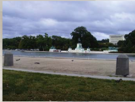
EXCESSIVELY SPACED BOLLARDS - PROVIDE NO PROTECTION
