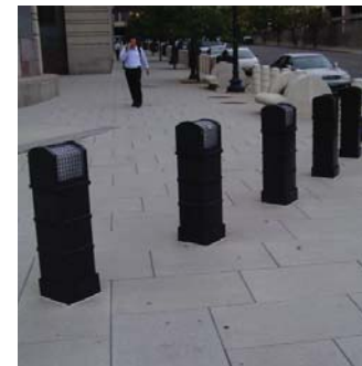
DESIGNED BOLLARDS AT ENTRY, THAT DOUBLE AS ILLUMINATION ELEMENTS AT NIGHT AND OTHER BOLLARDS MATERIAL, COLOR, AND DETAIL INTENDED TO BLEND INTO THE GROUND PAVING AND BUILDING ELEVATION RELATE AN ATTEMPT TO DESIGN BOLLARDS.
