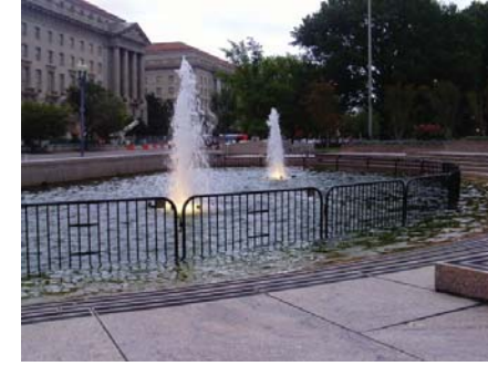
INSTALLATION OF PORTABLE FENCING, LIKELY INTENDED TO PREVENT PEOPLE FROM ENTERING THE FOUNTAIN, CLEARLY IS A FAILURE TO ENACT AN APPROPRIATE DESIGNED RESPONSE.
