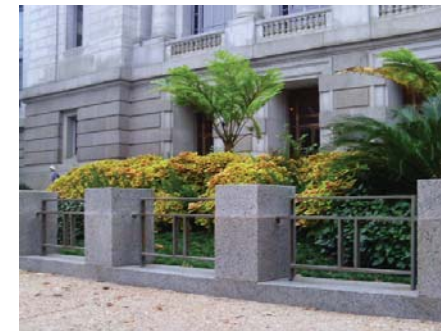
BARRIER OF CRENNELATED MASSES WITH CONNECTING METAL WORK SHOWS SOME RUDIMENTARY ATTEMPT OF COVERING BOLLARDS WITH SCULPTURAL DETAIL.
